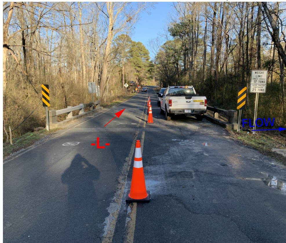
WEST APPROACH AT END BENT 1 LOOKING EAST
